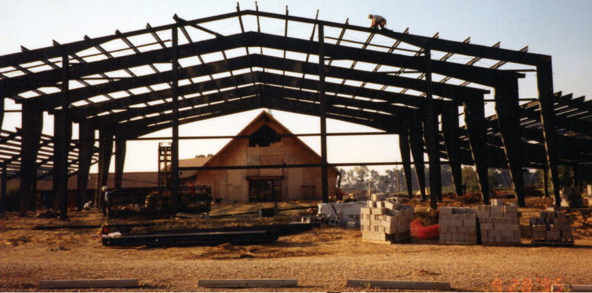
Construction of the Central Venue (originally known as the Worship and Activities Center (WAC))
