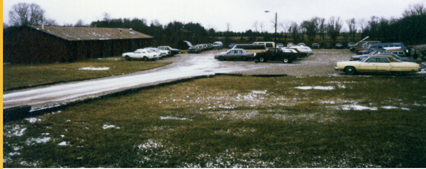
The first structure at the corner of Morse and Harrison (currently the Shalom Center).
